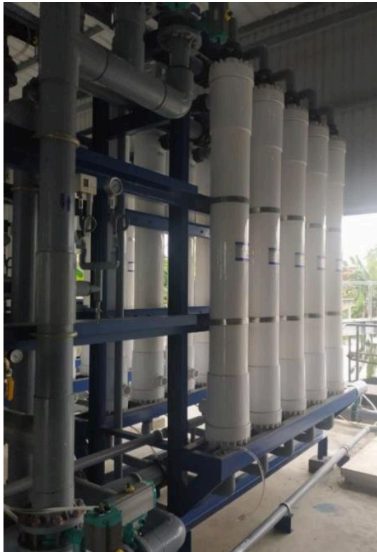
Figure 28. UF membrane system
