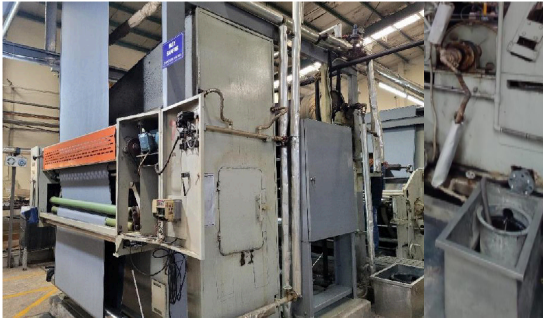
Figure 9. Post-cooling water of the Sanfor machine is filtered before being pumped to the cooling tower and recirculated to cool the machine
