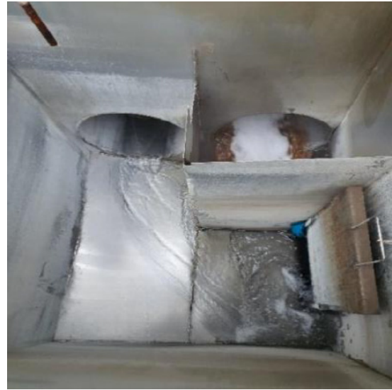
Figure 18. Dividing the discharge stream from the dyeing process at another factory
