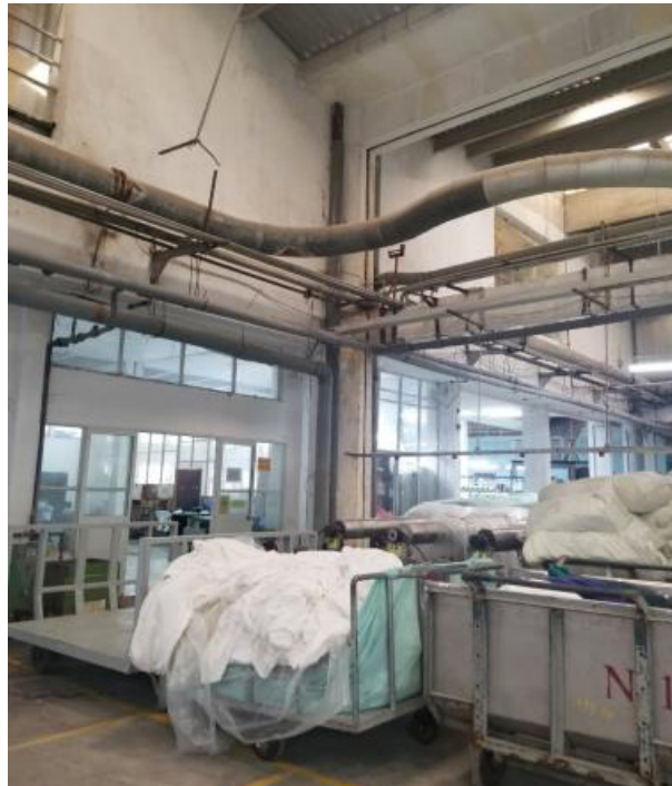
Figure 33. Rainwater pipeline system connected to drainage ditch
